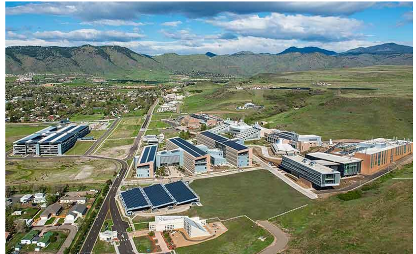
Net Zero Buildings at the National Renewable Energy Laboratory in Golden Colorado
